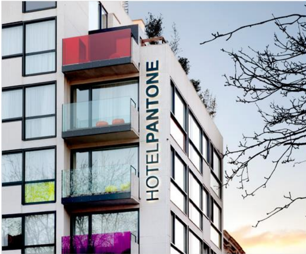
Figure 21. Base, Pantone Hotel, outside view.
