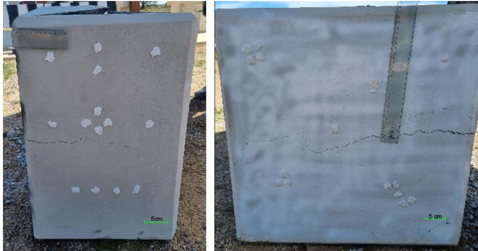
Figure 4.21: Visible cracks on the block after the impact.
