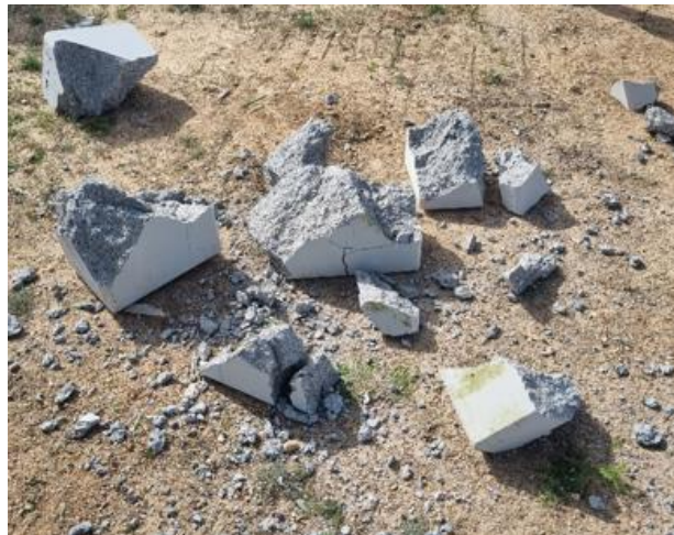
Figure 4.18: Display of the concrete block after the impact.
