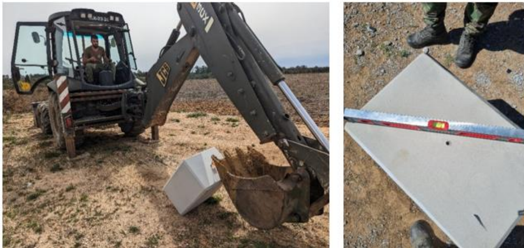
Figure 4.14: Process of the target placement.
