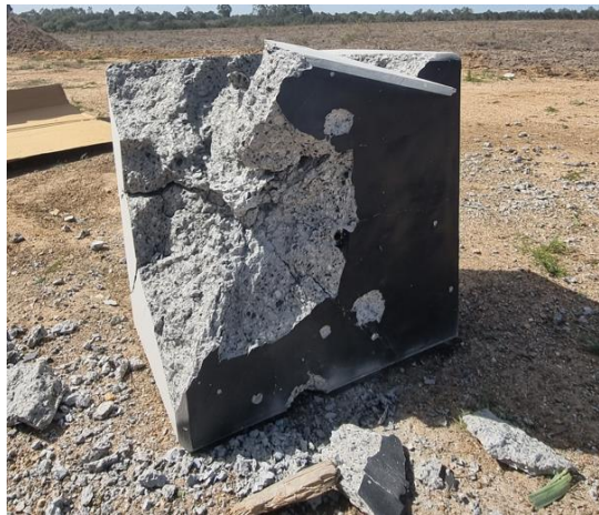
Figure 4.20: Block 2 after the impact.
