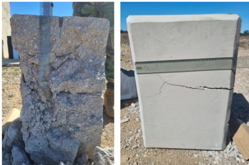
Figure 4.36: Damaged side of the concrete and the opposite side.
