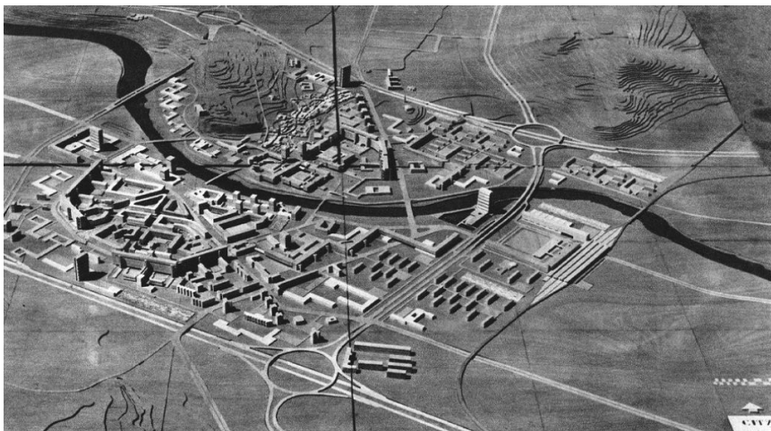
Figure 7. Johannes Van den Broek and Jacob Bakema, Competition design for the rebuilding of Skopje central area, 1965. Repro: Skopje resurgent: The Story of a United Nations Special Fund Town Planning Project . New York, United Nations Development Programme, 1970, p. 310.
