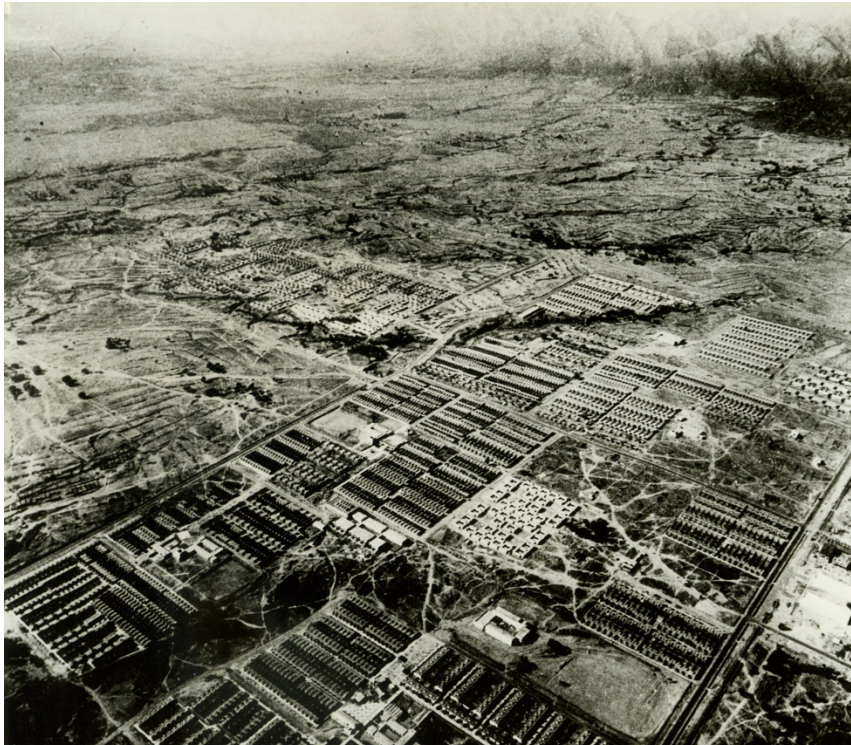
Figure 4. Aerial view of two sectors in Islamabad (G6-1 & G6-2). (Source: Constantinos A. Doxiadis Archives, © Constantinos and Emma Doxiadis Foundation)
