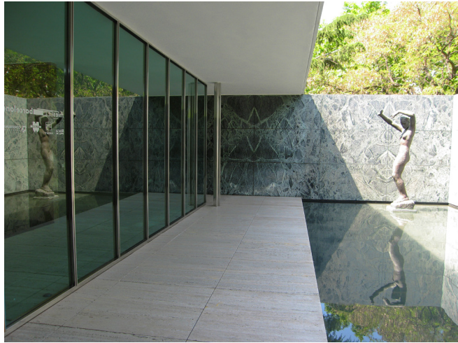
Figure 4. Detail of the combination of sandwich and megaron spaces in the Barcelona Pavilion, 1929. 'Mies van der Rohe'. Author's archives.
