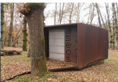
Fig.17: Vista general aseos
